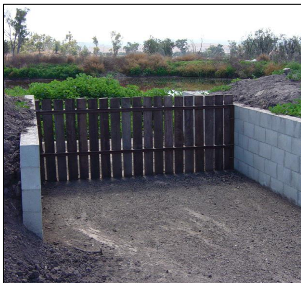
Figure 5: Typical sediment weir between sediment and effluent ponds
